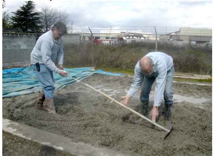
A 6" – 7" slump required an average of 20 pounds of pull force.
