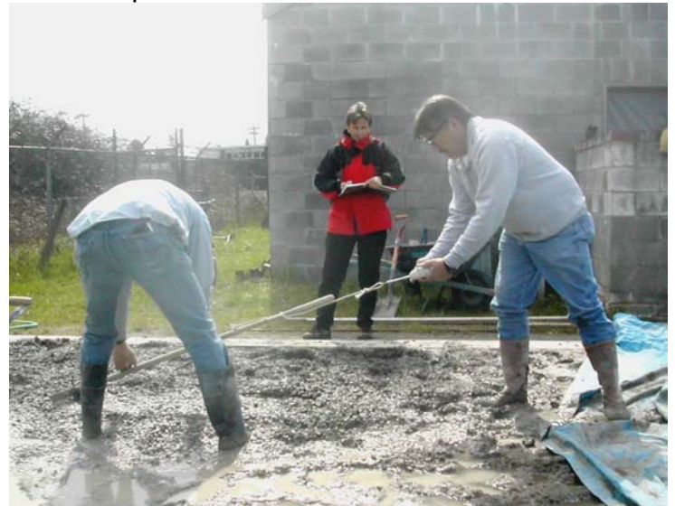
A 3" slump is measured here
